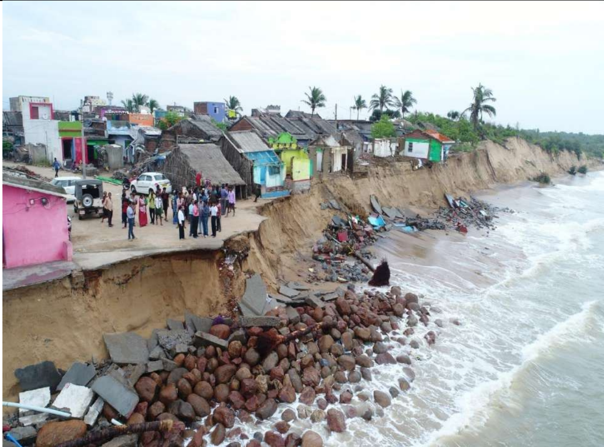
RAMAYAPATANA - Shoreline erosion during cyclone "Titili " on 11.10.2018
