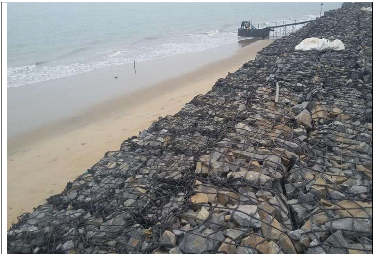
Accretion of sand has started in front of Geo Tube embankment at Pentha
