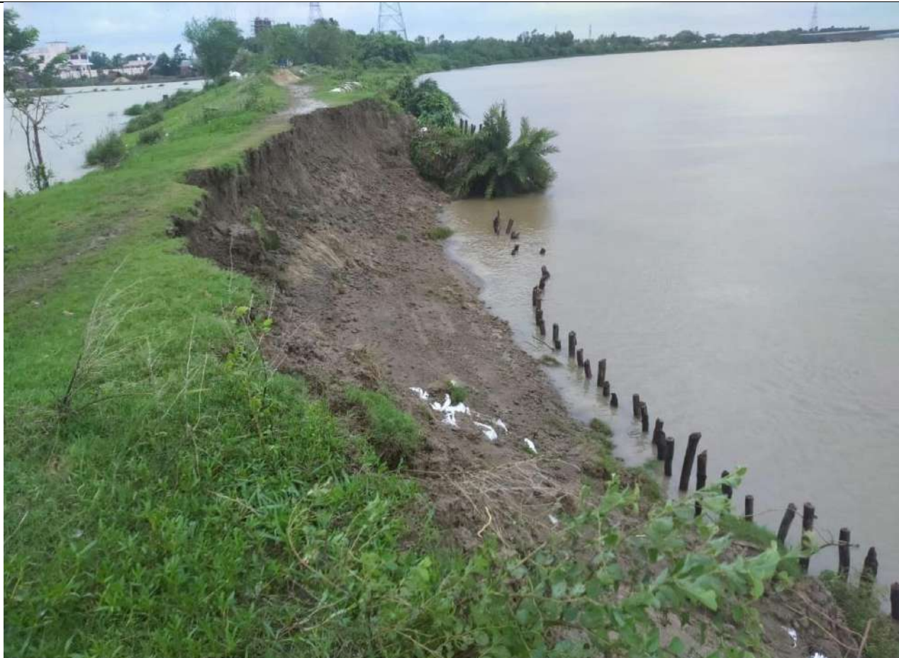
Damage of Keradagada Altnaga saline Embankment on Hansua right due to Cyclone "YAAS"
